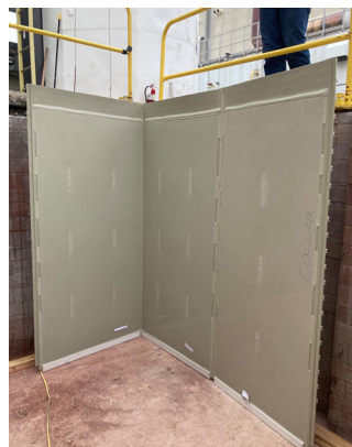
1. Project begins with corner dual wall sheet fitting - Note the existing red brick lining in background that was left in place.
