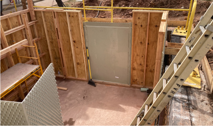
3. Additional forms are placed - Note the cavity between the ACROLINE liner attached to the concrete formwork and original masonry wall, visible behind the ladder at right.
