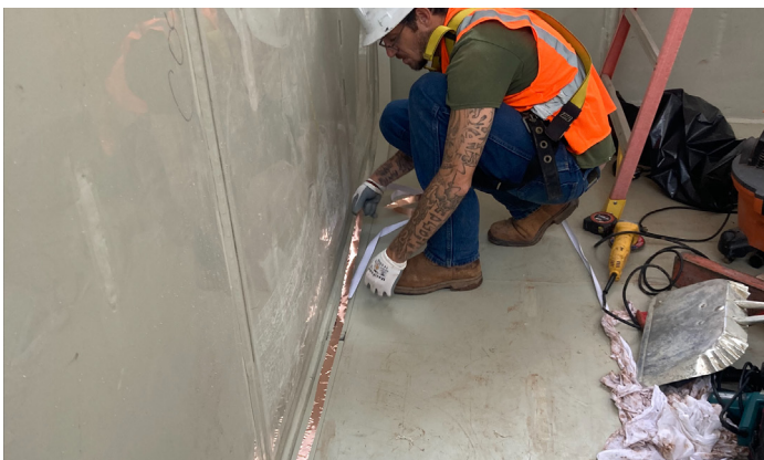
7. Conductive copper tape strips are added - Electrically conductive tape placed on top of the secondary liner before the primary liner is welded into place enable nondestructive holiday testing of the field welds.
