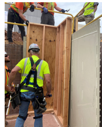
2. Custom fitted concrete wall forms installed - The concrete overpour cavity can be seen on the right edge of the picture.
