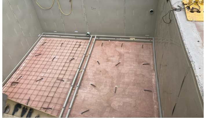
4. Floor preparation - Floor frames and wire mesh are installed with metal anchors to ensure proper grout anchoring and thickness.
