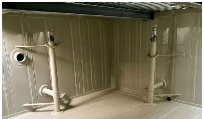
8. Work nears completion - Standpipes collect any liquid that leaks into the space between the primary and secondary liners.
