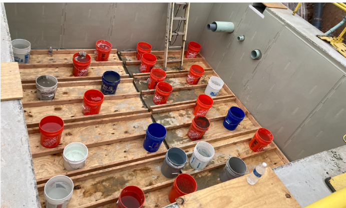
5. Floor installation - The installation of the floor proceeds after the walls have been installed. Special techniques are required to ensure the floor is properly fitted and grouted to achieve full contact.
